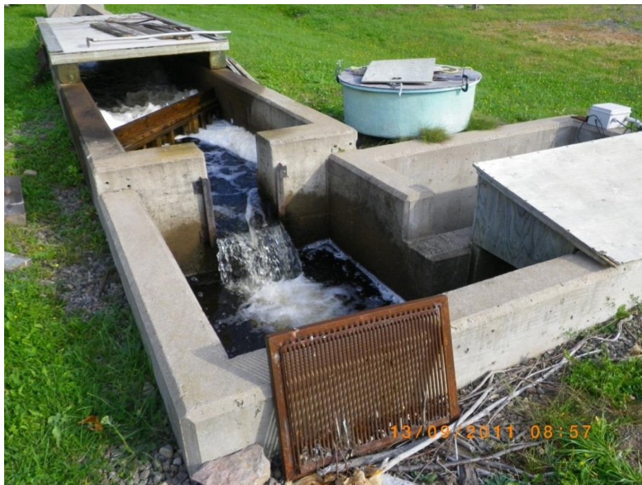
Figure 5.1. Bypass collection structure used during 2011 and 2012 to capture downstream migrating silver stage American eel from the Gaspereau River system at White Rock. The steel grate, located in the foreground, was installed nightly to collect eels within the lower concrete holding area. A green flow through circular tank, located in the background, was used to hold eels for approximately 24hrs post-surgery until release.
